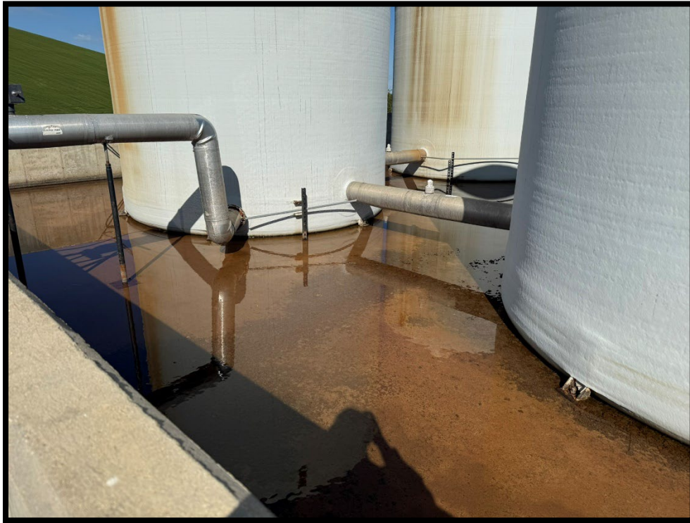
Photograph 1: View of minimal stormwater in containment.
