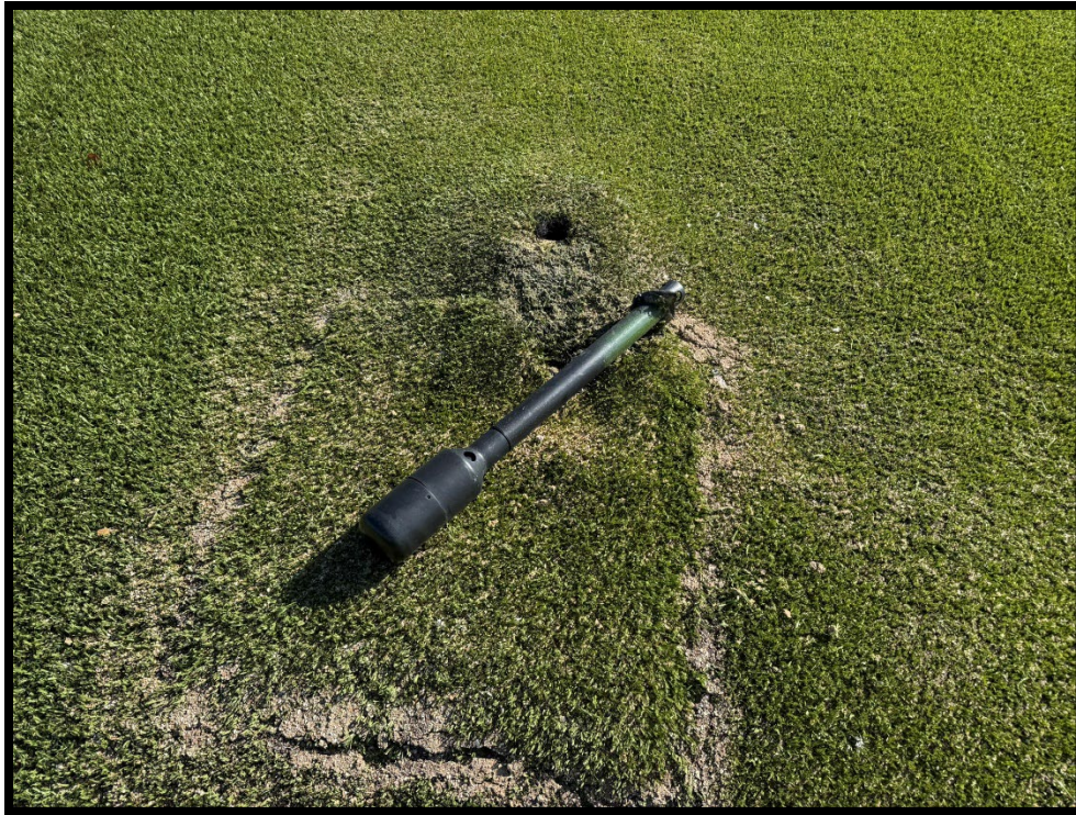
Photograph 3: View of damaged pressure relief vent on west side of Area 1-2.
